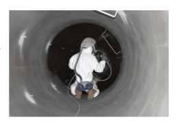
flanges are left unpainted, as the profile of the metal sprayed zinc aids the strength and friction of the bolted joints. There is an approximate curing time of two hours at 40 to 50°c. The mid-coat, commonly a 2-component high build epoxy, is then sprayed at around 120 microns DFT for the internal surfaces of the tower and 150 microns on the external surfaces.
