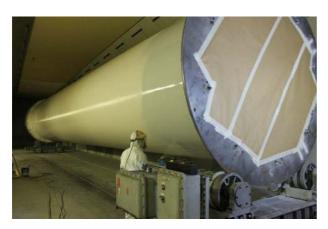
There is a further two hours curing time required at 40 to 50 °c. The final top coat to be applied is around 50 microns DFT of 2-component gloss acrylic polyurethane to the external surfaces of the tower. There is approximately four hours curing time required at this stage, again at 40 to 50 °c.
